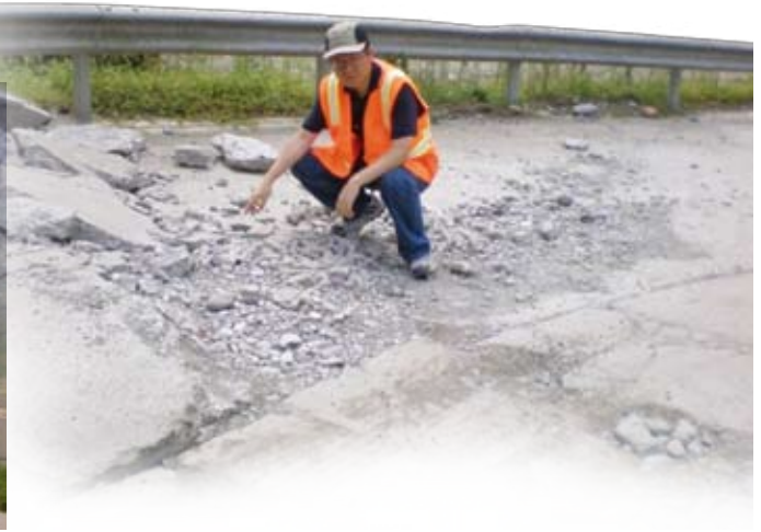
Investigating the damage to the road.
